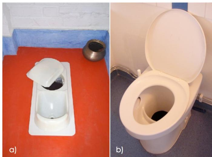
**Figure 3: a) a urine-diverting dry squat toilet from India (photo: S.Vishwanath [www.rainwaterclub.org](http://www.rainwaterclub.org)); b) a urine-diverting dry toilet from Sweden (photo: Dana Cordell).**
