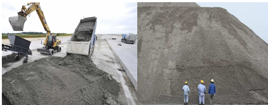
Concrete sludge: a waste generated in construction sites. Steelmaking slag: a byproduct in the iron and steel industry.
